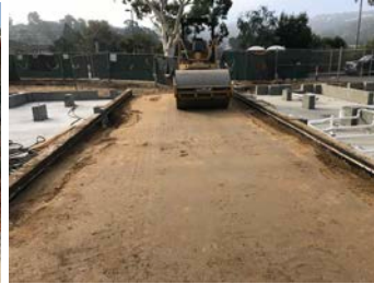
Site work at CLC
