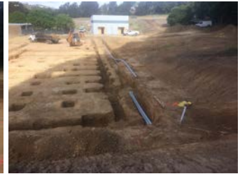
Grading and footings underway for new CLC classrooms
