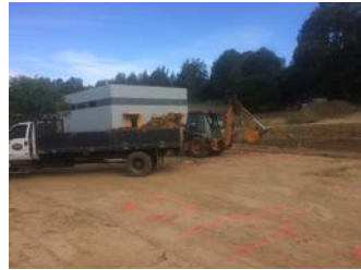
Grading and footings underway for new CLC classrooms
