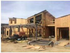
Steel and Framing at New Learning Commons
